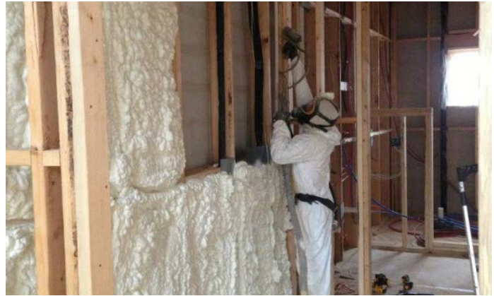
Enertite open-cell spray foam being installed by Vis Viva Energy & Services
