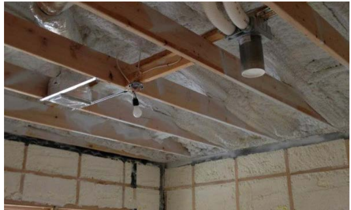
Complete building envelope sealing with BASF Enertite
